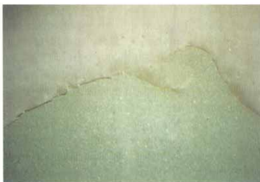
b. The cement was mixed under vacuum.
