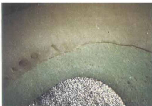
a. The cement was mixed at atmospheric pressure.
