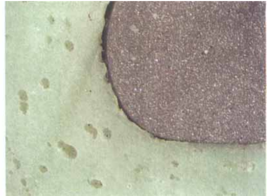
b. The close-up shows a gap with "saw tooth" edge at the cement-stem interface.
